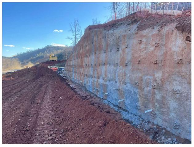
Complete soil nail installation and temporary shotcrete facing
