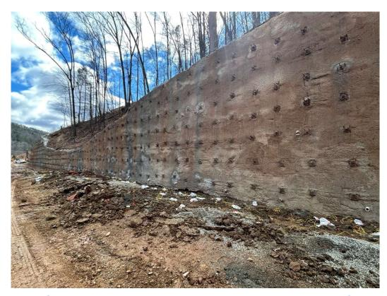
Complete soil nail installation and shotcrete facing
